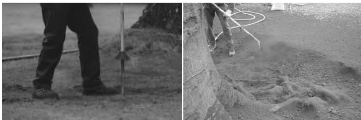
Fot. A i B. Rozluźnianie gruntu w technol. AirSpade [źródło: Technical Applications Bulletin use of compressed Air-powered Excavation for Arboricultural Site Works, AirSpade Technical Applications Bulletin]
